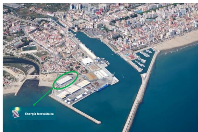
Figure 5: The solar energy plant located in shed 4 of the Port of Gandia
