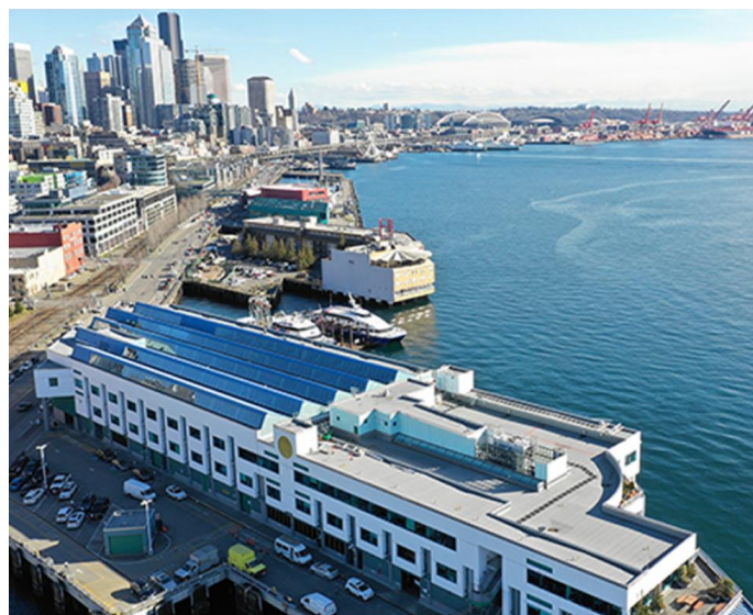
Figure 31: Pier 69 Solar Project
