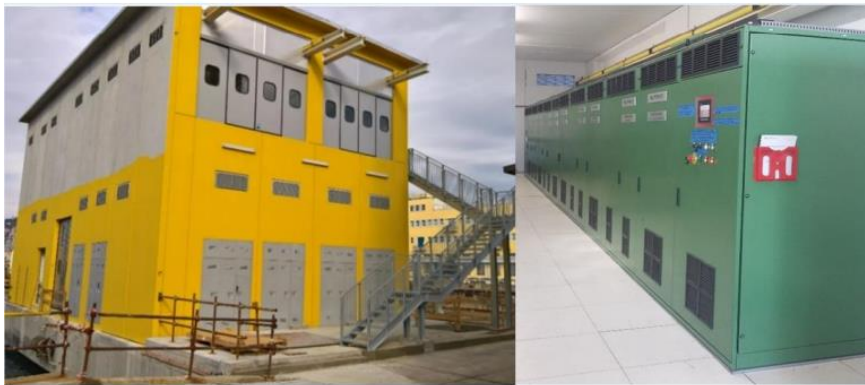
Figure 17: The stations and sub-stations of OPS facilities for ship repair areas in Genoa
