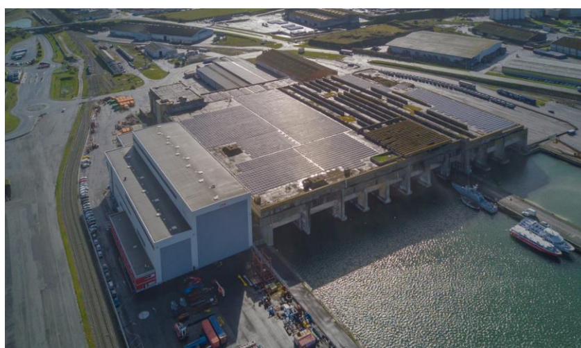
Figure 20: The roof of the submarine base in the La Rochelle port
