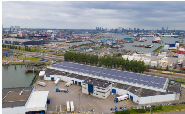
Figure 8: Largest solar panel system in the Rotterdam port
