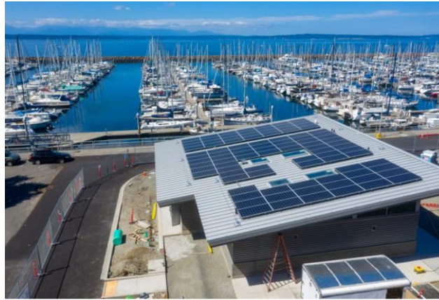
Figure 33: Shilshole Bay Marina Solar Project 57
