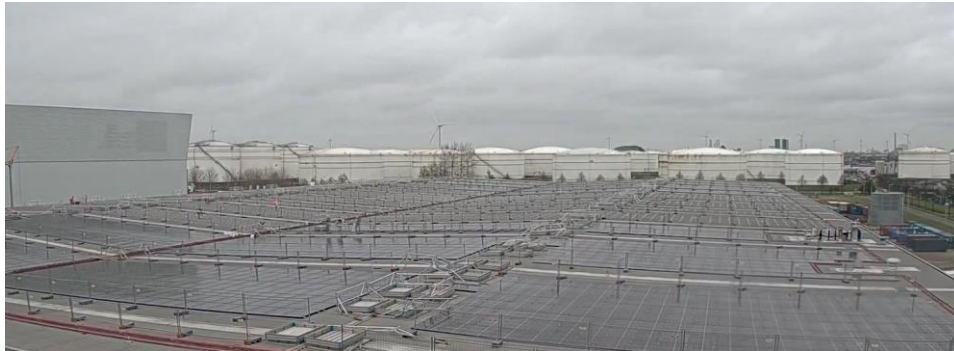
Figure 10: Solar installations in the port of Amsterdam 21
